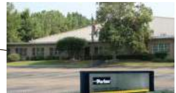
Fluid Control Division Facility, Madison, MS.
